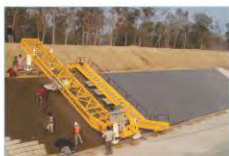
Concrete Canal Paver
